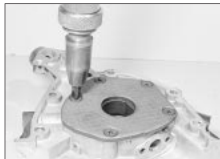
14.1 Using an impact screwdriver to undo the oil pump rear cover screws
